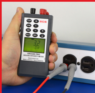
Measuring Ohm Impedance between Neutral and Ground
